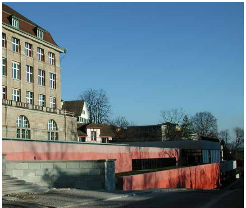
Below: Retaining wall for a subterranean auditorium at the University of Zurich (2002), Gigon Guyer
